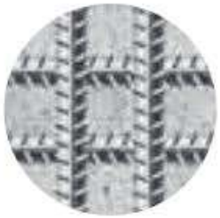
Highly reinforced concrete
